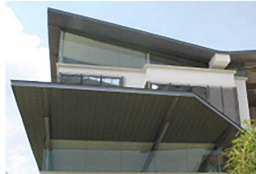
Linearform panel is used as the soffit ceiling at private bungalow in Kuala Lumpur
